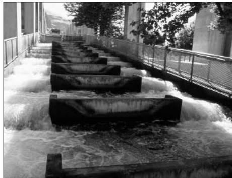
Current FERC relicensing rules allow dam operators to challenge agency required fish protections such as fish ladders. Photograph by Jim Yuskavitch
