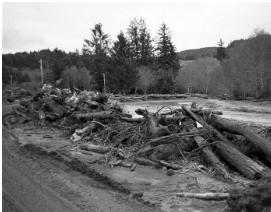
A major blow-out in November 1999 on "Doug's River" shows the destructive power of a culvert failure. Photo by Doug Schaad
