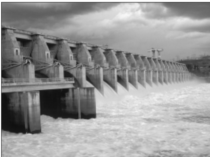
Drought conditions in 2001 wreaked havoc for fish and people alike across the Pacific Northwest from the Klamath basin (top photo) to the Columbia River. Photos by Jim Yuskavitch
